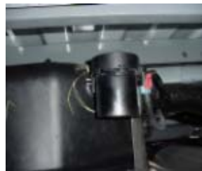
Figure C1, Step 1: Locate the Fuel Valve.
