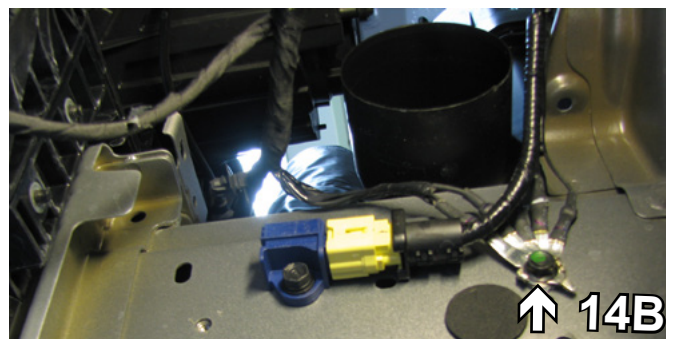
14. On the driver side, using a 10MM socket remove the ground wires from the left side and reattach them with the ground wires on the right side.
