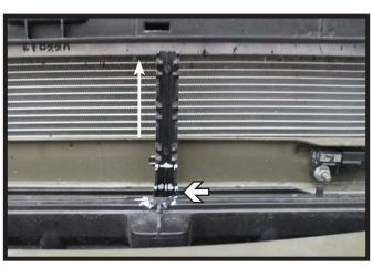
13. **SFE Models:** Pull up on the shutter rod. Trim off the rod flush with the base for baseplate clearance.
